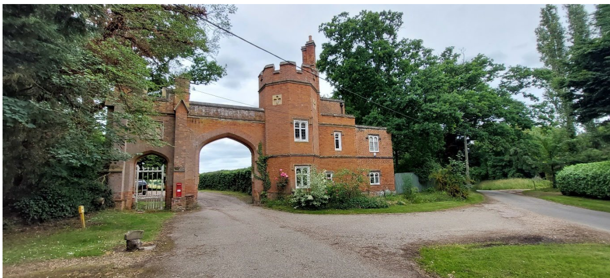
Figure 3: Gate and lodge at entrance to former Edwardstone Hall
