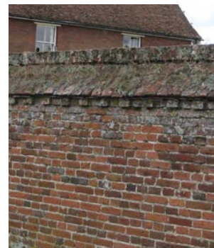
Red brick wall with saddleback brick coping
