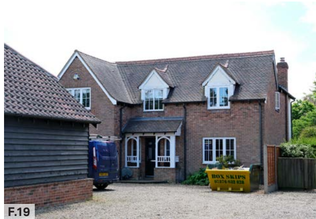
Figure 19: A two-storey dwelling with a mixed red brick facade and clay tile roofing.
