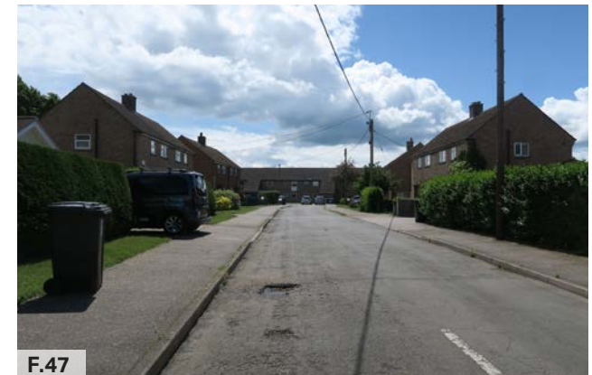
Figure 47: Photo of a more recent development in Mill Green with footways on both sides of the carriageway.
